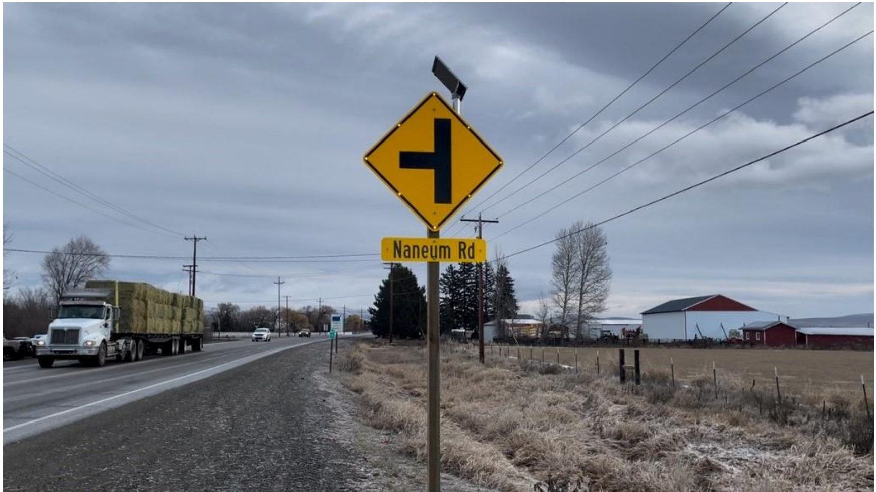
Naneum Rd LED Intersection Warning Sign
