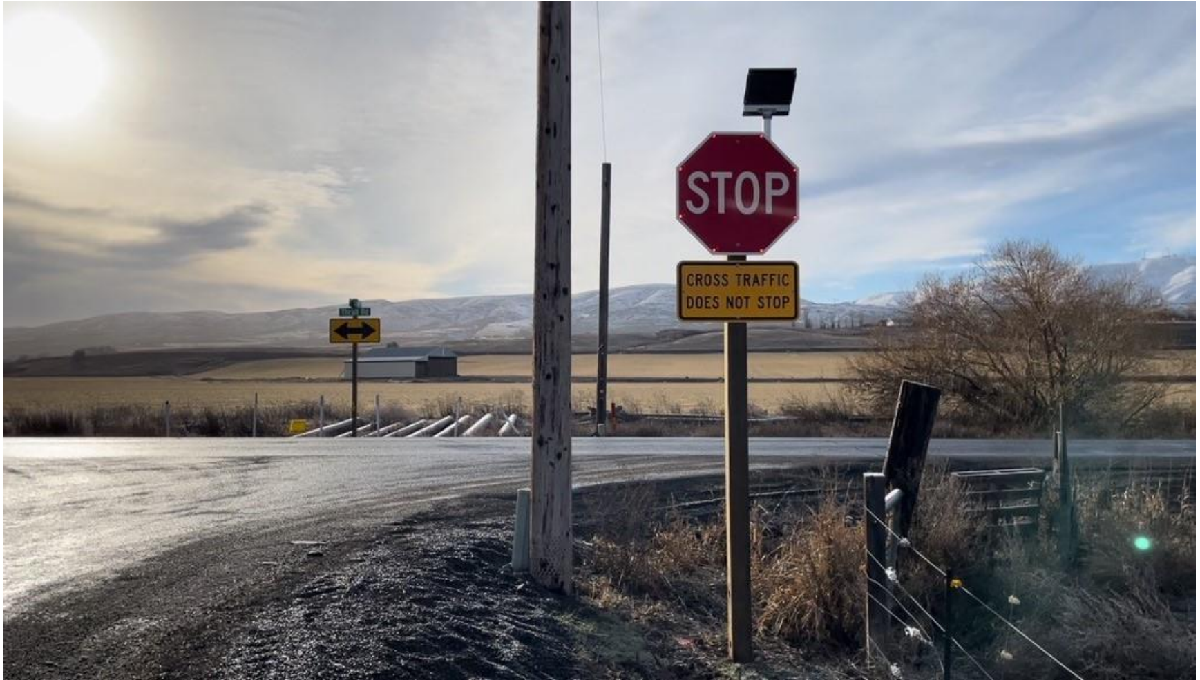
Clemens Rd LED Stop Sign
